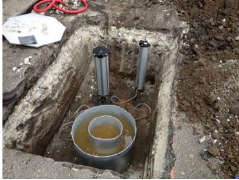
Figure 13. Double-ring infiltrometer test per ASTM D3385.
