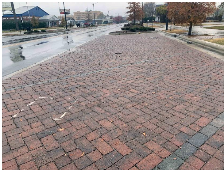
Figure 1. PICP in Fayetteville, NC. This pavement was cleaned after 6 years of service. The white marks are where infiltration test was conducted to assess cleaning results. The marks will fade with time.
